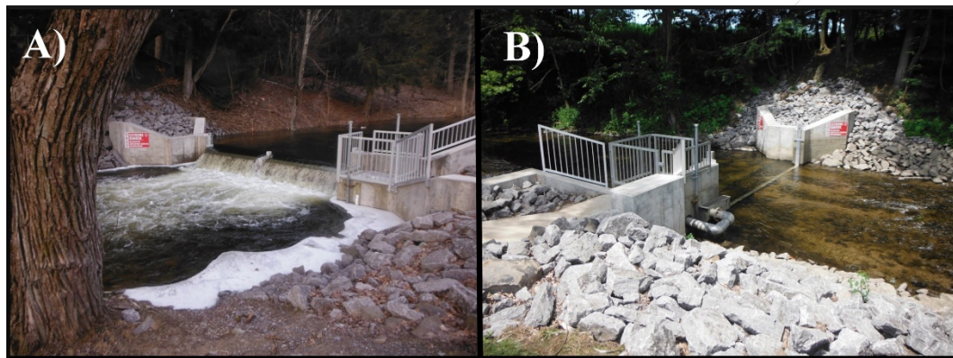
Figure 4-2. Example of a manually operated seasonal-barrier in Orwell Creek, tributary of the Salmon River, NY, with (A) stoplogs installed during sea lamprey migration and with (B) stoplogs removed. Photos courtesy of Fisheries and Oceans Canada.
