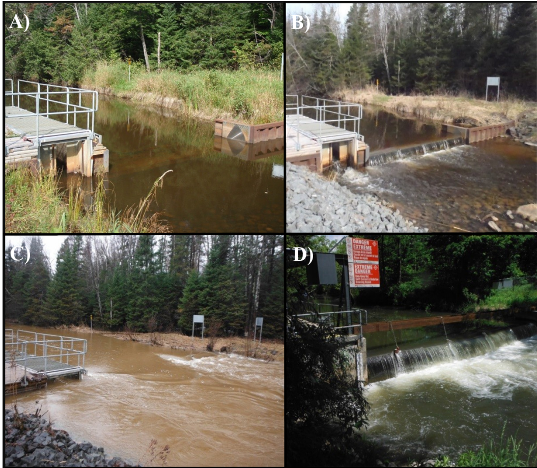
Figure 4-4. Big Carp River, ON (Lake Superior) inflatable crest barrier, (A) not operating with inflatable barrier down, (B) in the operating position with inflatable barrier raised, (C) inflatable barrier raised during flooding, and (D) beam used to lift the inflatable-crest barrier when the computerized control system failed at the barrier on the Big Creek River, ON (Lake Erie). Photos courtesy of Fisheries and Oceans Canada.
