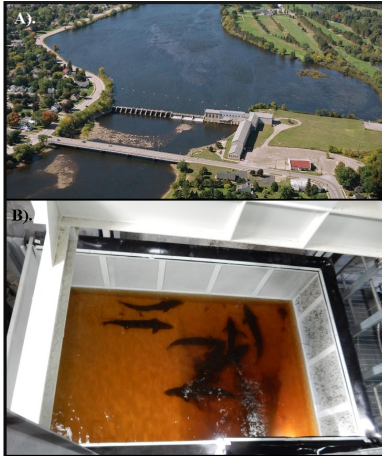
Figure 2-2. (A) Menominee/Park Mill Hydroelectric Project on the Menominee River, MI (Lake Michigan). (B) Fish elevator raising lake sturgeon into sorting facility for processing. Grating on the elevator was sized to reduce capture of sea lamprey. Lake sturgeon are manually sorted and transported upstream via truck. All remaining fish are released downstream of the dam. Photos courtesy of the U.S. Fish and Wildlife Service and Eagle Creek Renewable Energy.
